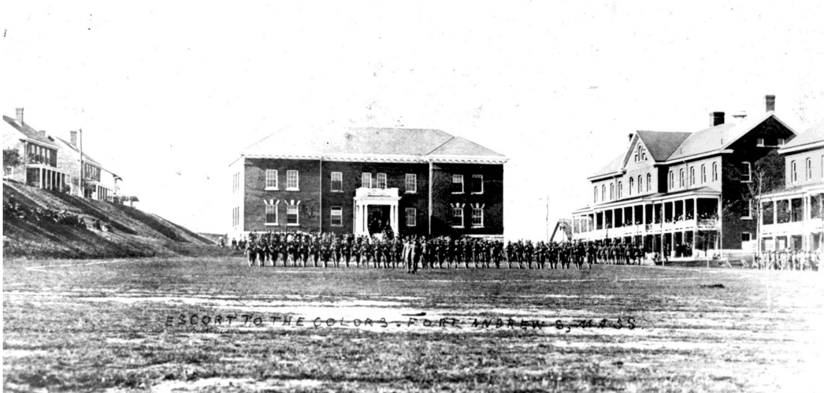
Figure 14. View looking northwest from the parade ground to the administration building (#26), after 1912. At image left are steps to officers' quarters (#s 15,14,34) and at image right are barracks (#s 10,11). Young trees and steps are faintly visible in front of the barracks. (DCR 2009: 49)
