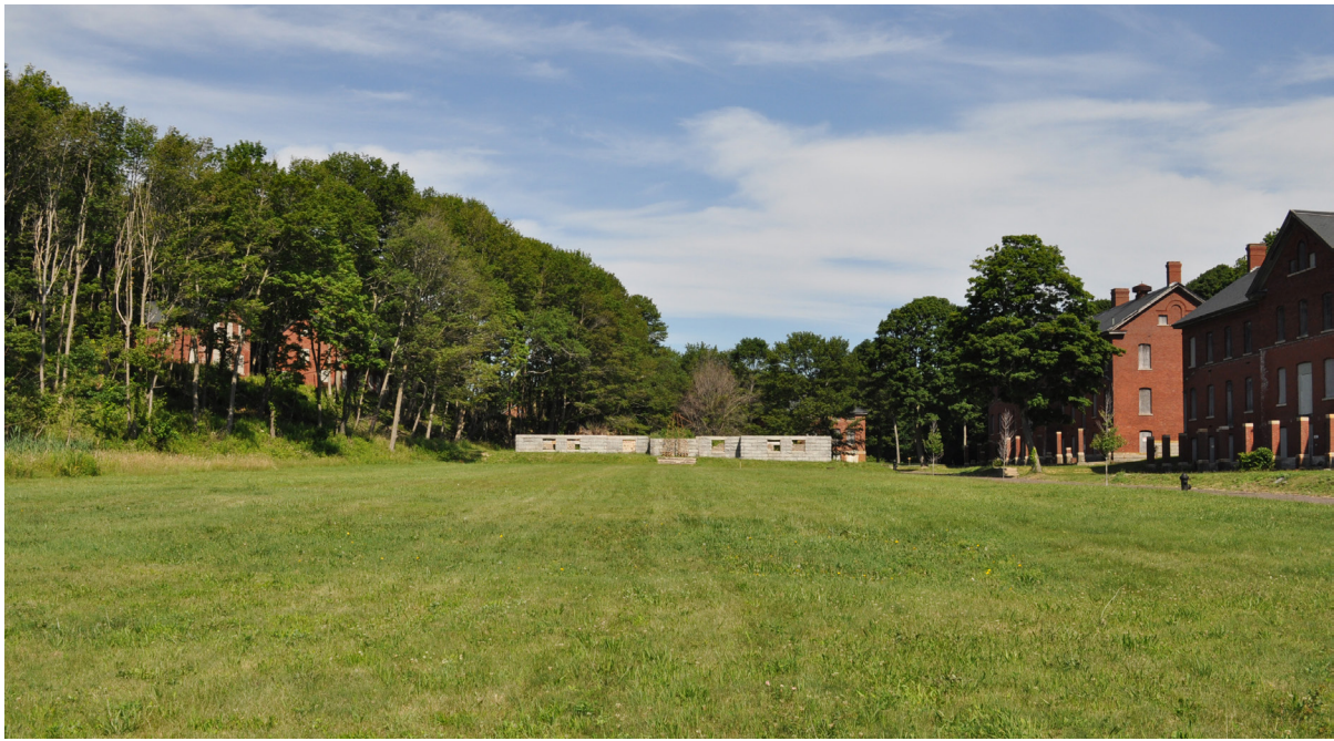
Figure 63. The historic view from the parade ground has been restored, and compares well with the scene in Figure 14. View looking west. (OCLP 2017, DSC-0429)
