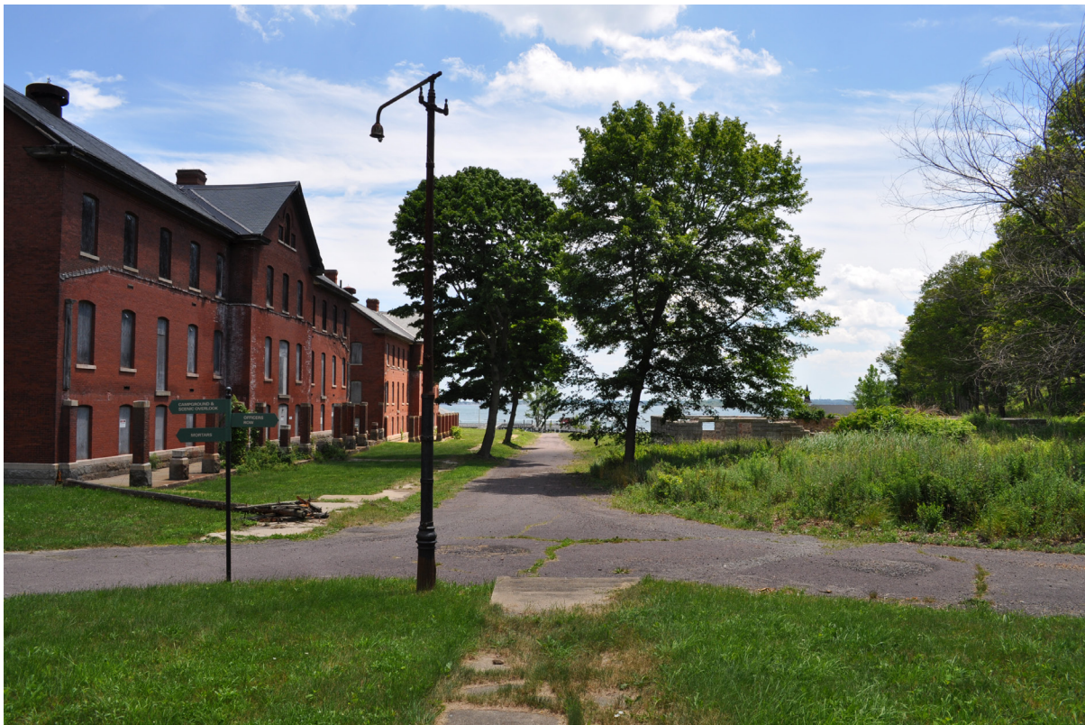
Figure 67. A historic light pole still stands in front of the recreation hall. View looking east. (OCLP 2017, DSC-0549)
