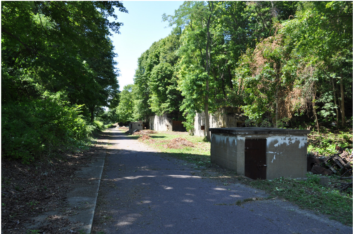
Figure 40. The orthogonal layout of the main road, sidewalk, and two mortar batteries contrasts with the curved layout of facilities along Officers' Row. View looking northwest. (OCLP 2015, DSC-0572)
