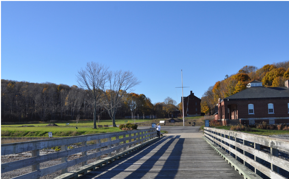
Figure 68. View of the flagpole at Fort Andrews. View looking west. (OCLP 2014, DSC-5471)
