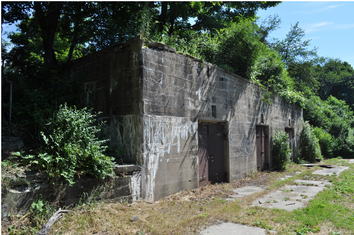
Figure 46. Overgrown vegetation on the rear elevations of Battery Bumpus and the two other gun batteries are mostly clear, but other components are cloaked in trees, shrubs, and vines. View looking northeast. (OCLP 2017, DSC-0458)
