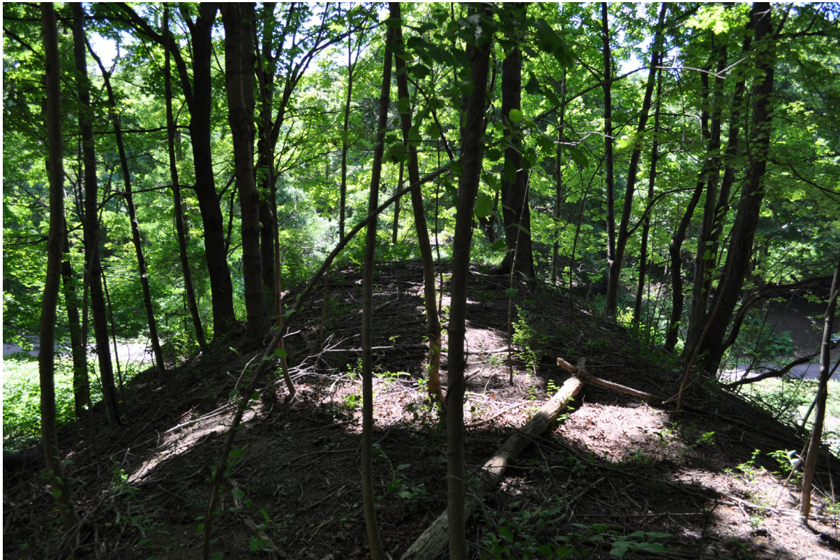
Figure 37. The contours of earthen embankment between the two mortar pits at Battery Cushing are still visible. View looking southwest. (OCLP 2017, DSC-0575)
