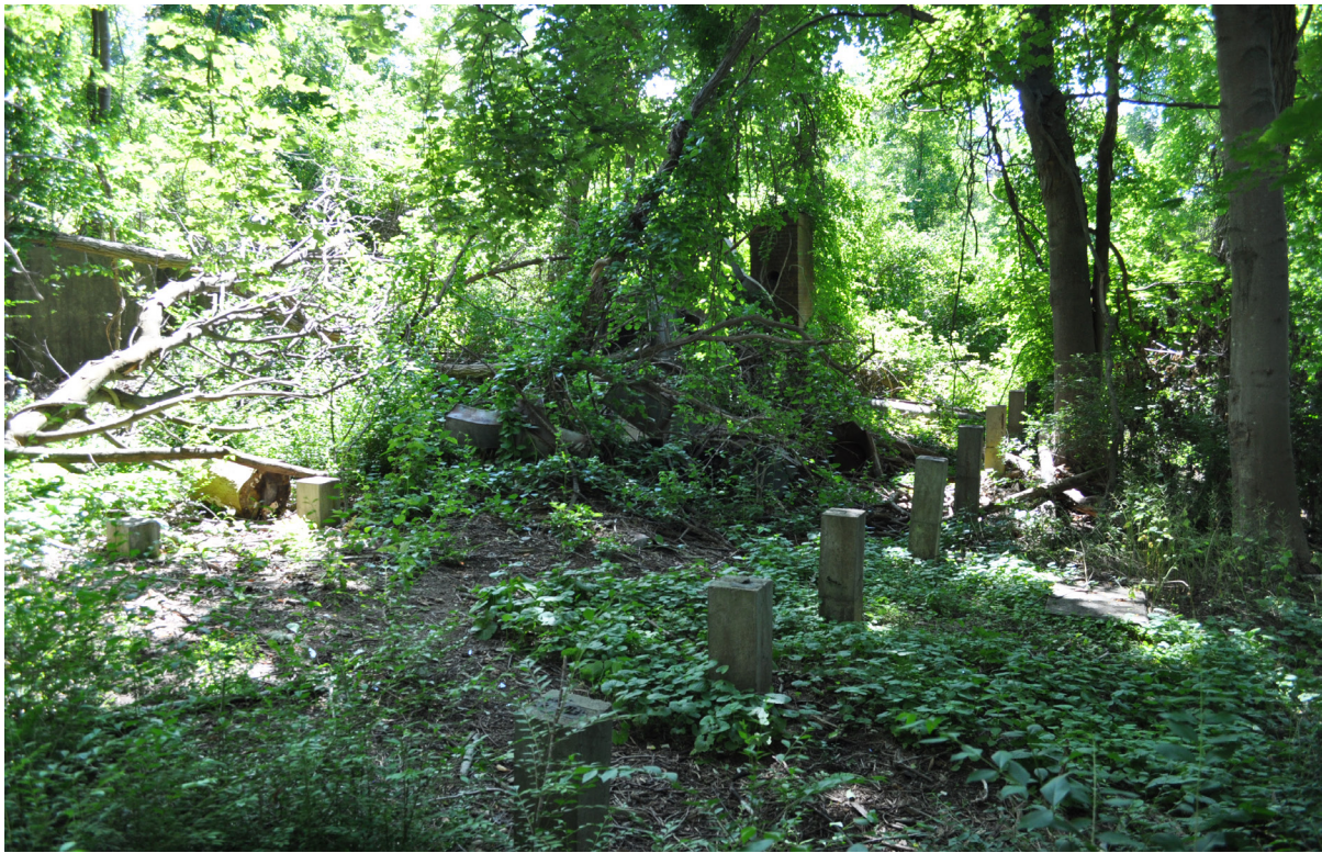
Figure 57. Concrete foundation posts, a brick chimney, and debris remain from a World War II-era temporary day room (#T-24) on the south drumlin. One of the concrete retaining walls built in this area is visible at image left. View looking west. (OCLP 2017, DSC-0724)
