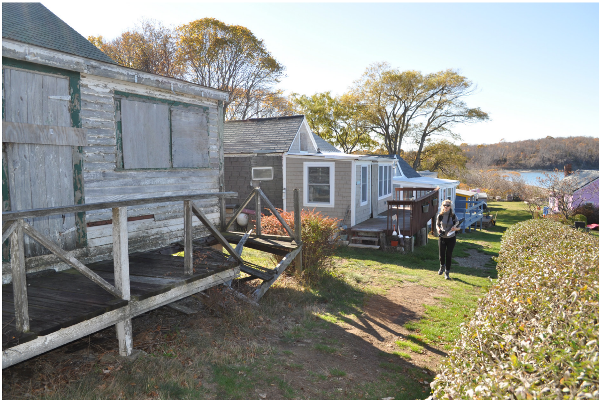
Figure 41. Row of cottages (#s 22, 23, 24, 25) facing northwest, on the northwest side of Middle Head. View looking southwest. (OCLP 2016, DSC-0460)
