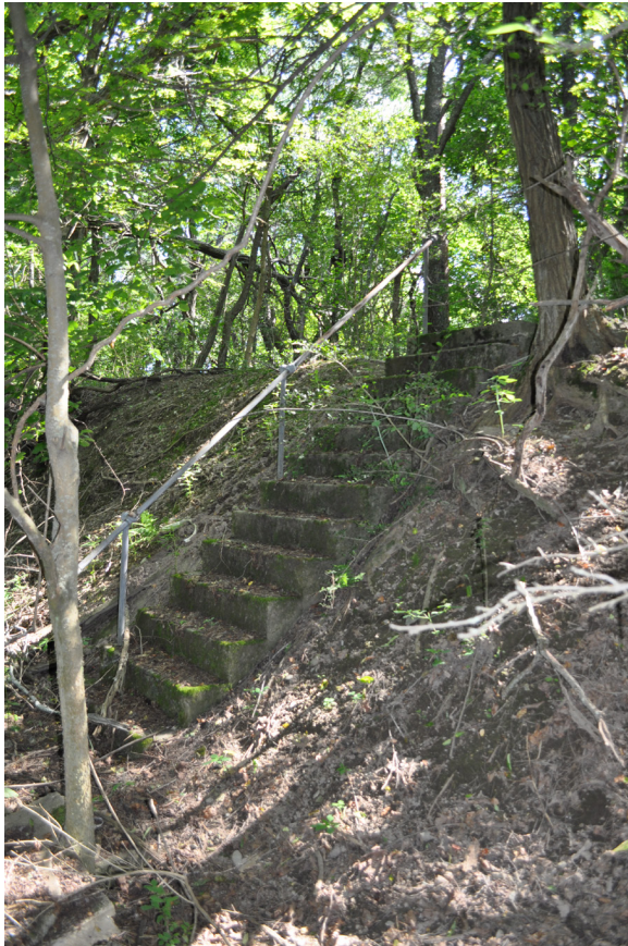
Figure 51. The only intact circulation feature at the top of the south drumlin is this staircase that accessed the ruins of the below-grade battery command/fire control structure (#F-105). View looking southeast. (OCLP 2017, DSC-0772)
