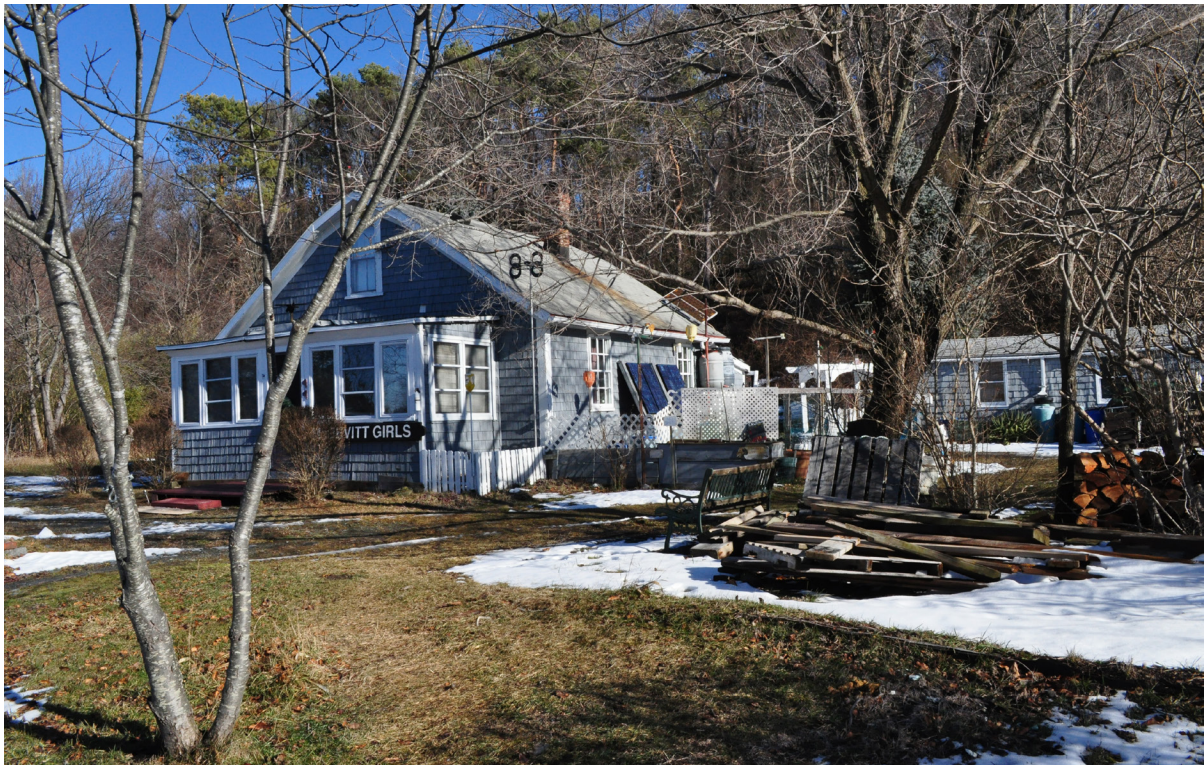
Figure 34. Cottage #44 is the last occupied building on Sergeants’ Row, built by a fort sergeant in the 1920s and now occupied by the McDevitts. View looking northeast. (OCLP 2015, DSC-6369)
