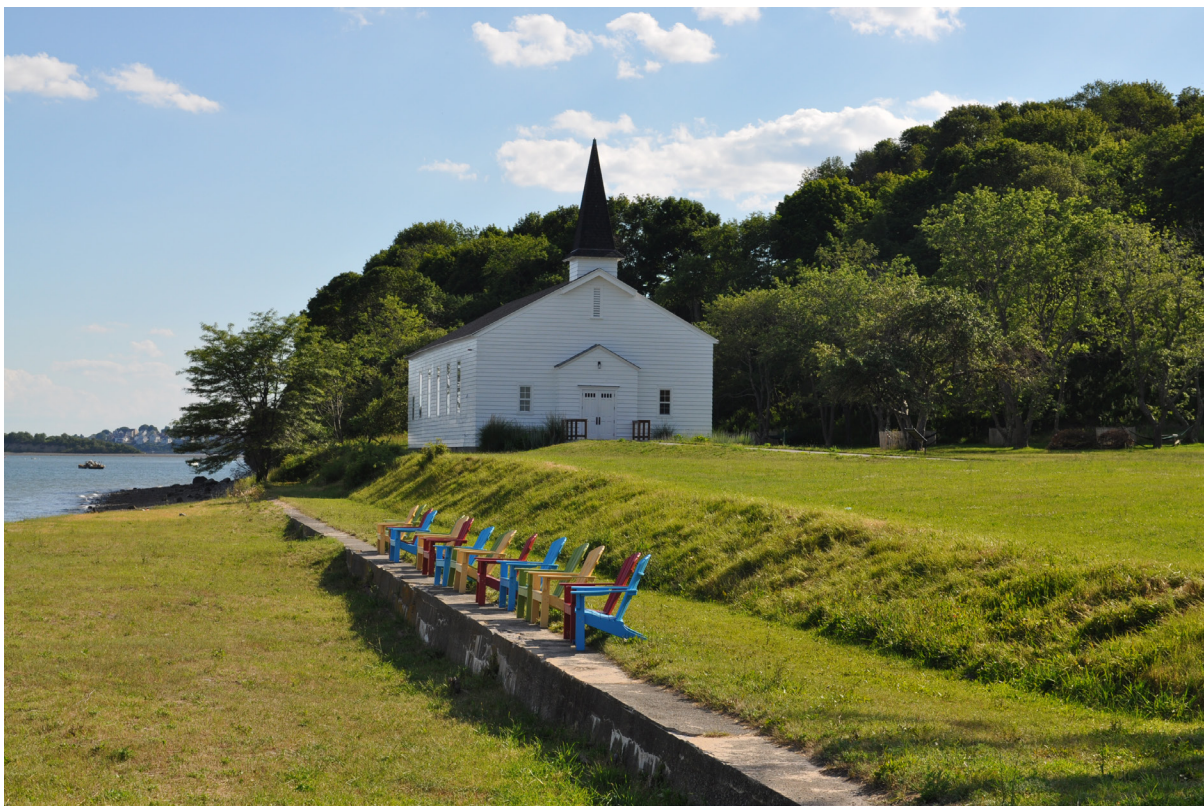
Figure 47. The chapel (#T-31) is fronted with new plantings, and a representative apple orchard stands just to the west. The 1912 army seawall (#48) is in the foreground. View looking southwest. (OCLP 2017, DSC-0849)
