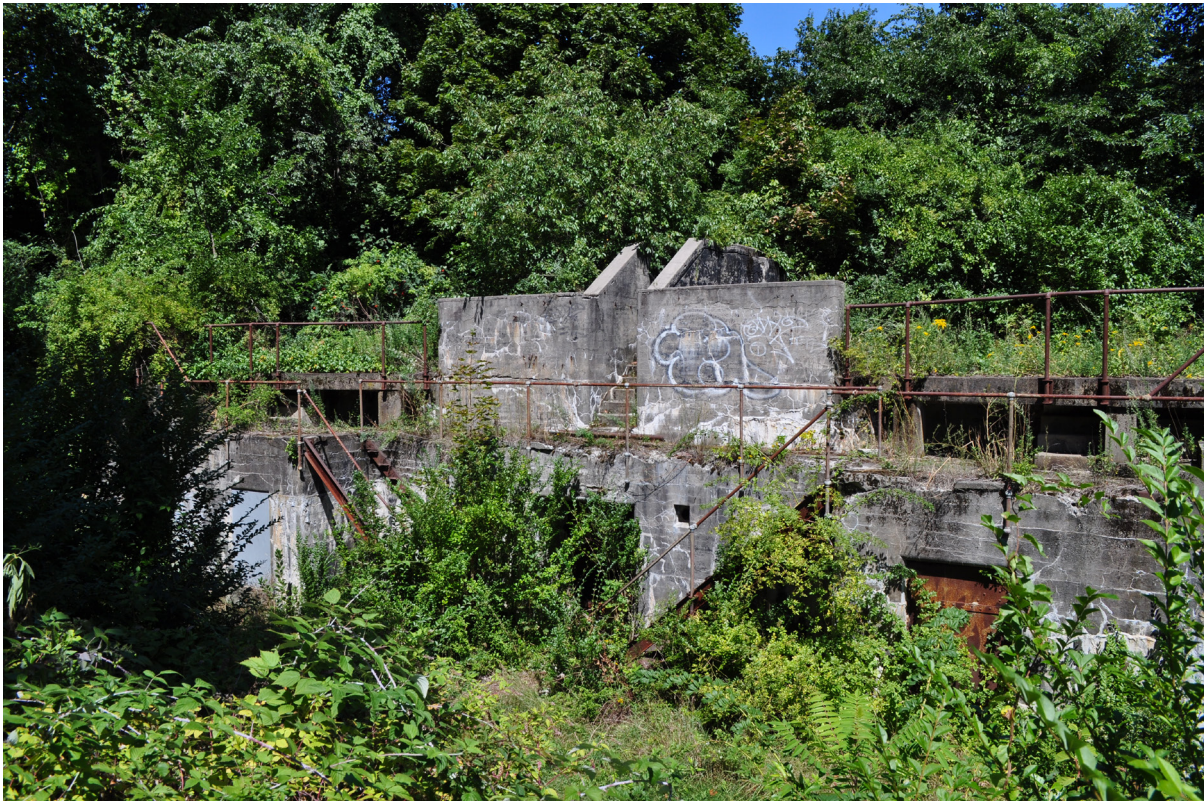
Figure 60. Vegetation envelops much of Battery McCook, built in 1901-04. View looking northwest. (OCLP 2014, DSC-0096)
