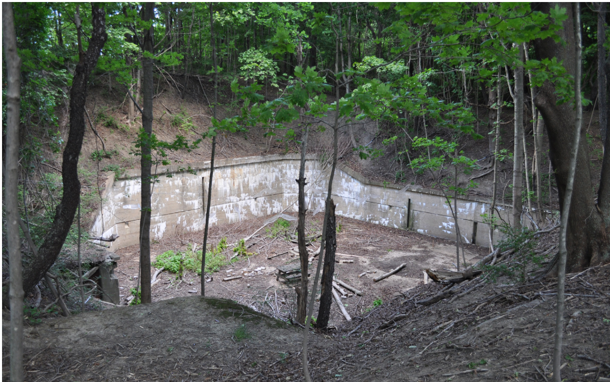
Figure 45. The park has cleared woody vegetation in the north mortar pit of Battery Whitman. View looking east. (OCLP 2017, DSC-0676)
