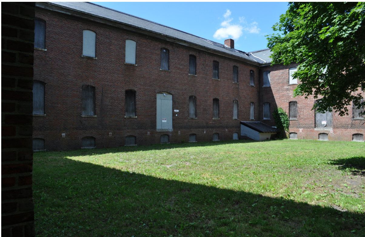
Figure 54. The U-shaped quartermaster storehouse (#36), the largest building at the fort, has been stabilized for future use. View looking north. (OCLP 2017, DSC-0705)
