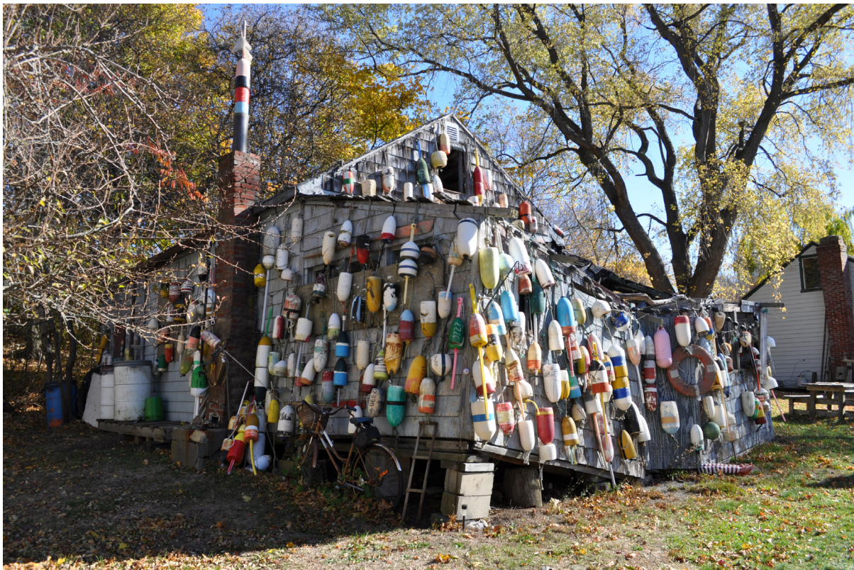
Figure 53. The decorated ruins of Cottage #32 on Crab Alley, Middle Head. View looking southeast. (OCLP 2016, DSC-0399)
