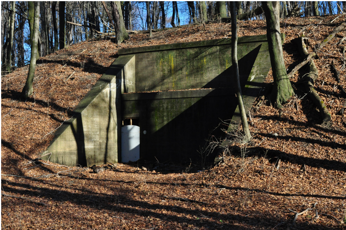
Figure 61. The concrete ordnance storehouse was built into the north drumlin in 1906. View looking north. (OCLP 2015, DSC-6339)
