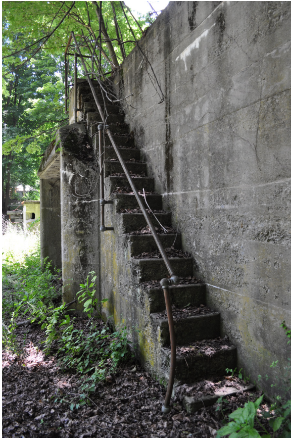
Figure 59. Stairs and railings in varying conditions remain throughout Battery Cushing, built in 1901-04. View looking southwest. (OCLP 2017, DSC-0614)
