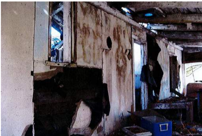
Interior condition of front porch, Cottage 39.
