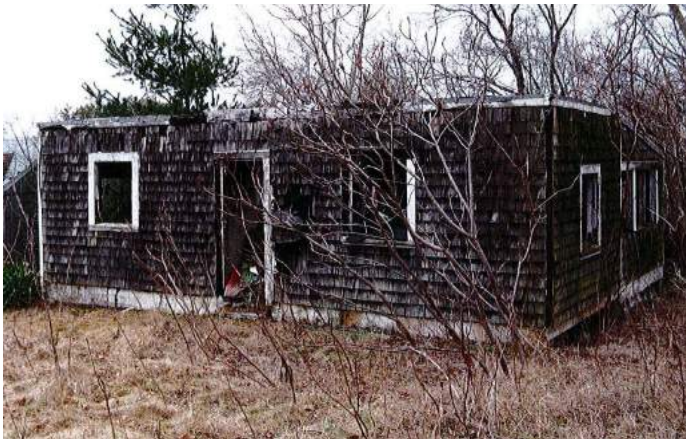
Cottage 39 entrance from NE.
