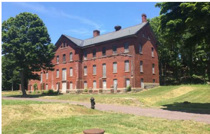
Building 11 from Parade Ground.
