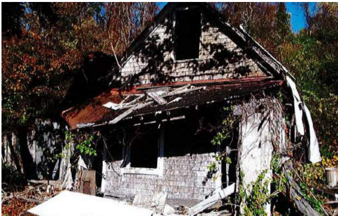
Enclosed entry porch W. elevation of Cottage 46.
