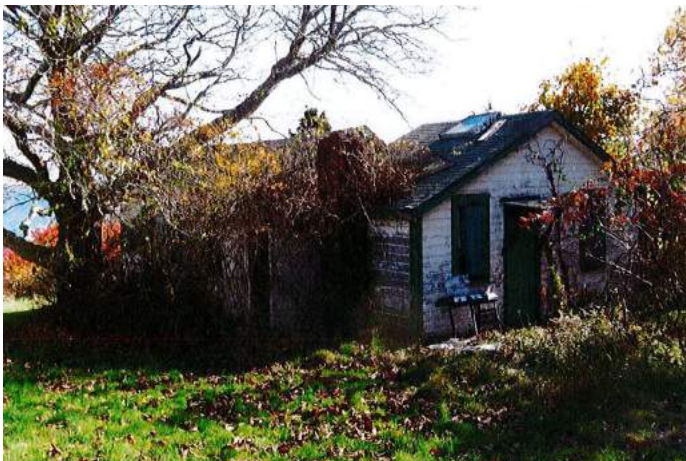
Cottage 06 from SW..
