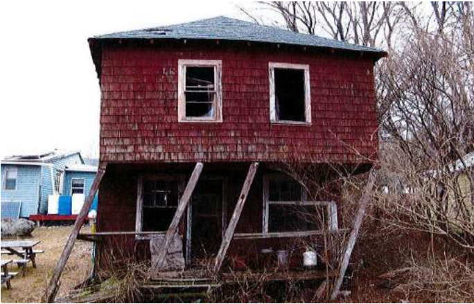
W. Overhang & porch, Cottage 28.
