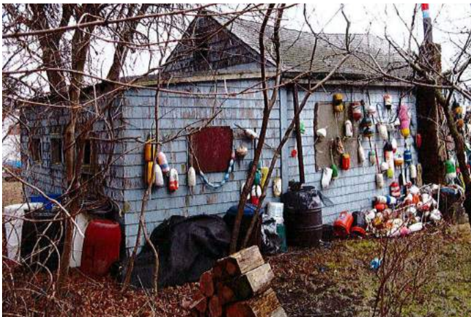
Rear extension Cottage 32.
