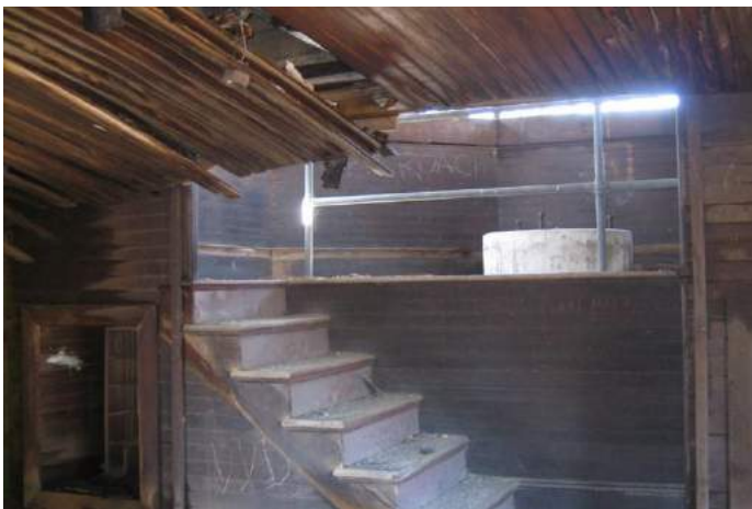
Building T2 Interior looking N.
