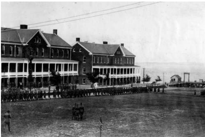
View of demolished Barracks adjacent to Building 10..
