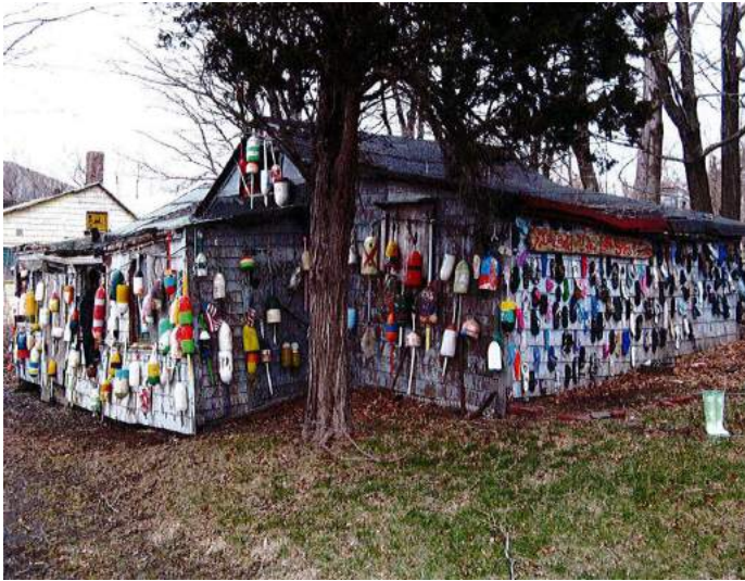
Cottage 30 from SW.
