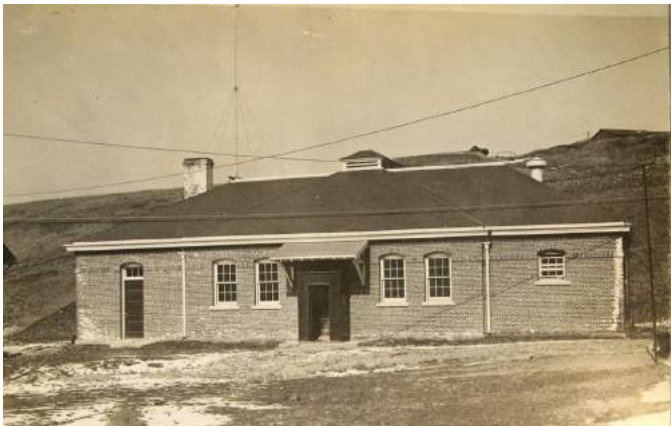
Building 08 from S. with Bldg. 33 to left. Historic view of Building 08.
