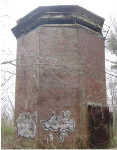
Fire Control Tower N. elevation.
