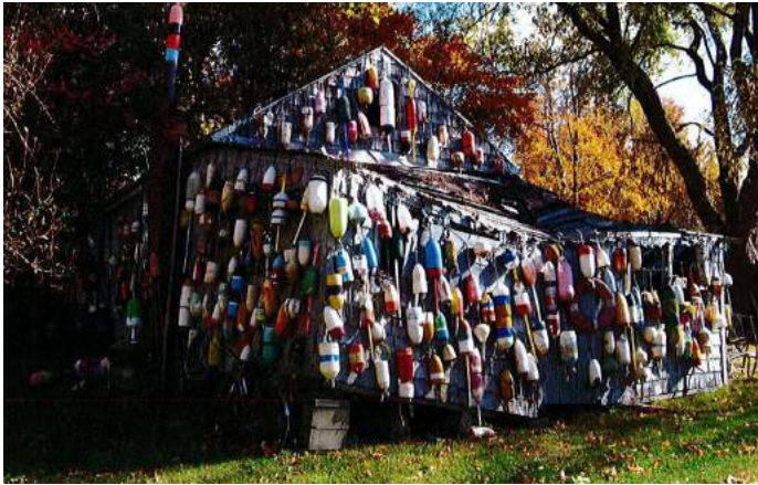
W. elevation Cottage 32 showing buoy decoration.
