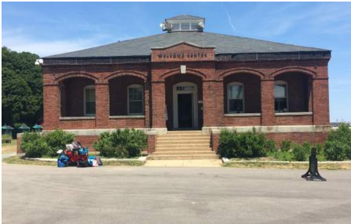
Front elevation of Building 31.
