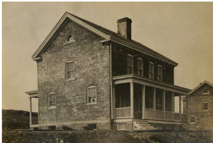
Historic view of Building 27 from NE corner.
