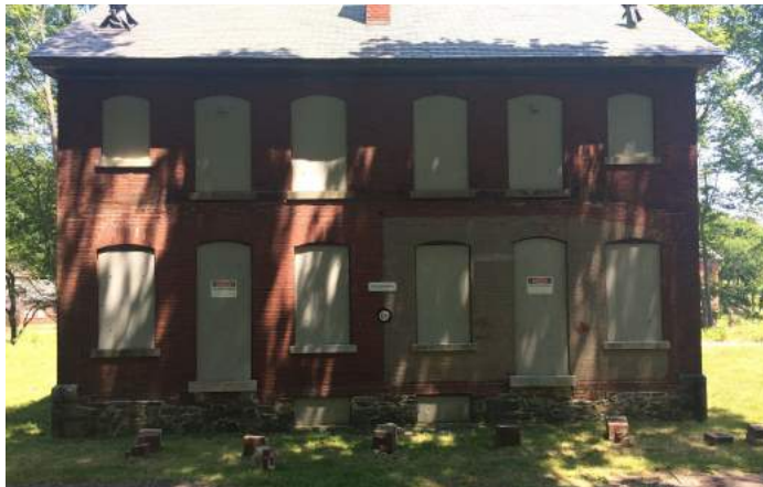
Building 15 S. elevation today.
