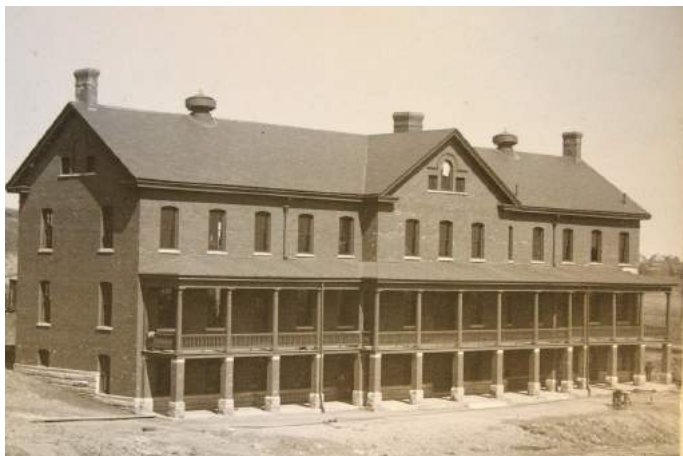
Covered porch Building 11, S. elevation.
