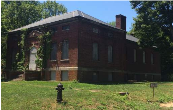
Gymnasium from NE corner.
