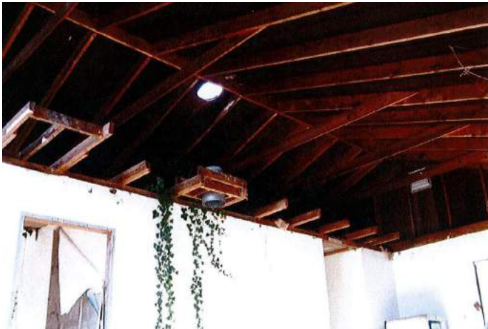
Interior of Cottage 09 showing cut back joists.
