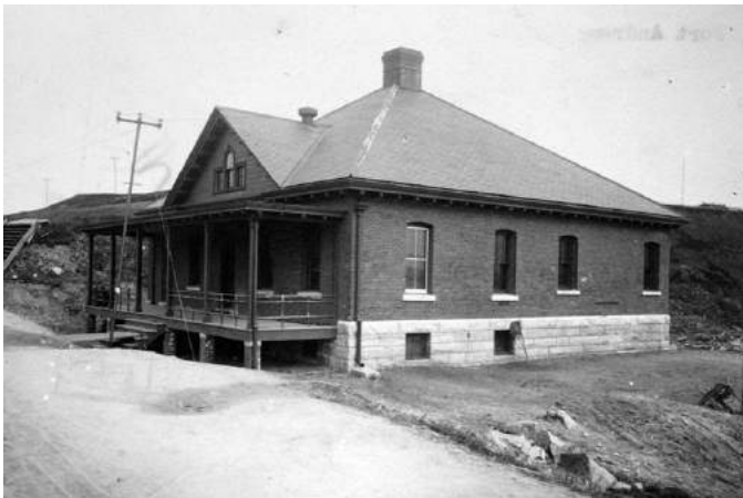
Original entrance to Building 07 S. elevation
