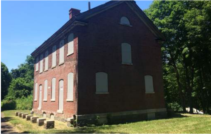
Building 28 looking W.
