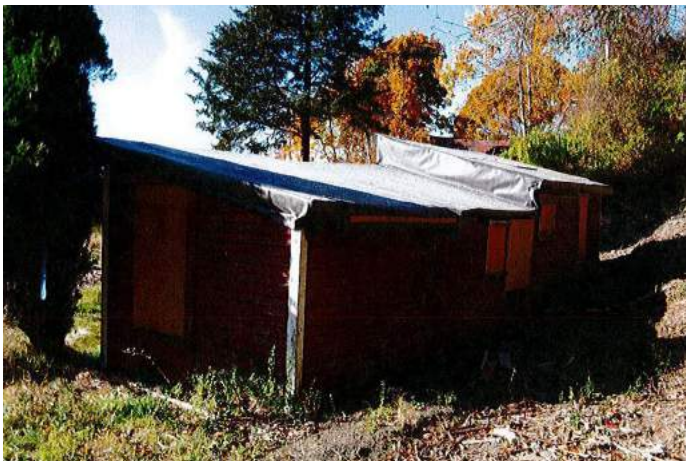
Temporary roof sheathing, Cottage 45.
